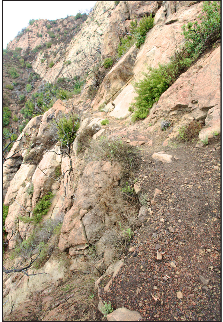
This part of the trail is extremely dangerous as it meanders across the front side of the Mission Crag. Adding additional crib walls and reinforcing existing ones will help
